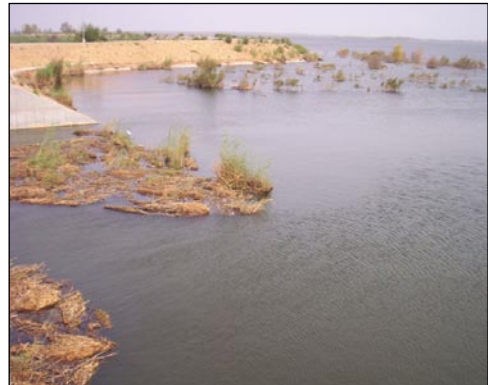
Photo 4. Chotiari reservoir outlet (Bakar lake area).
